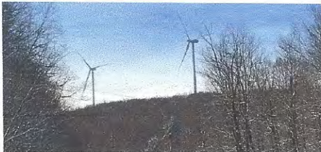
Wind farm near Altoona, Pa. | © RTO Insider
